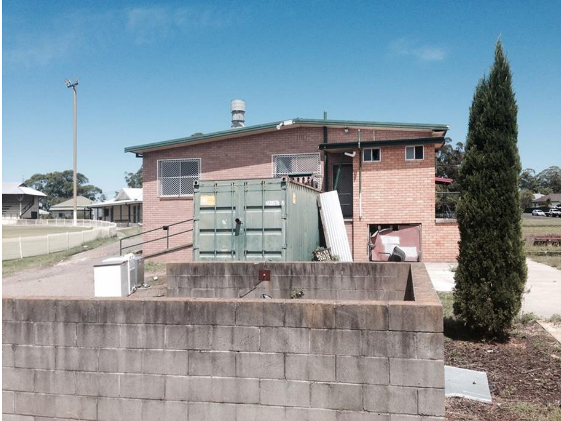
Photo 11 – Rear of former bowling club building
